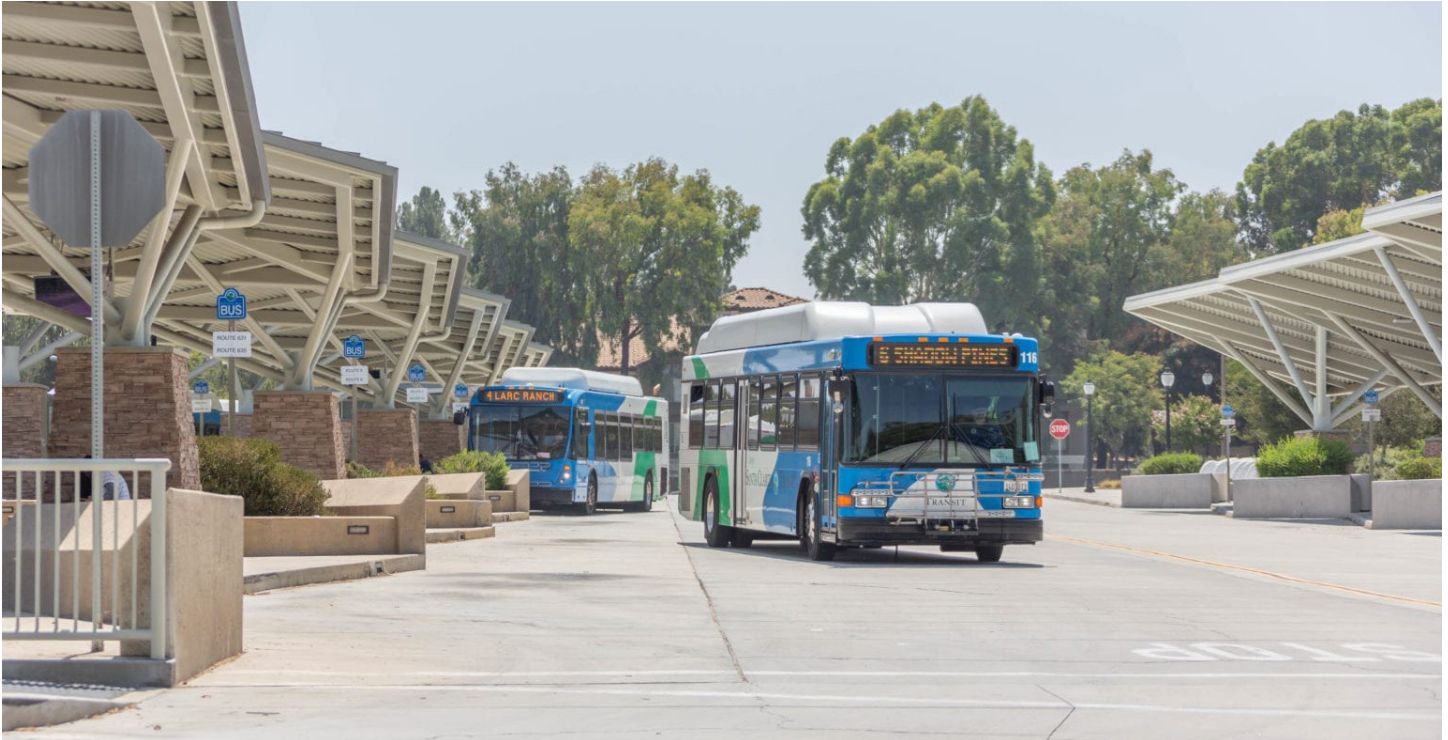
Figure 63: A bus leaving the McBean Regional Transit Center
