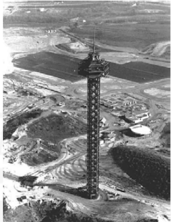
Construction of Magic Mountain-circa 1971
