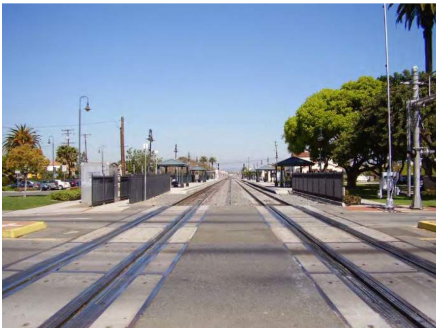
Figure 3-33. Stations near a Highway-Rail Grade Crossing
