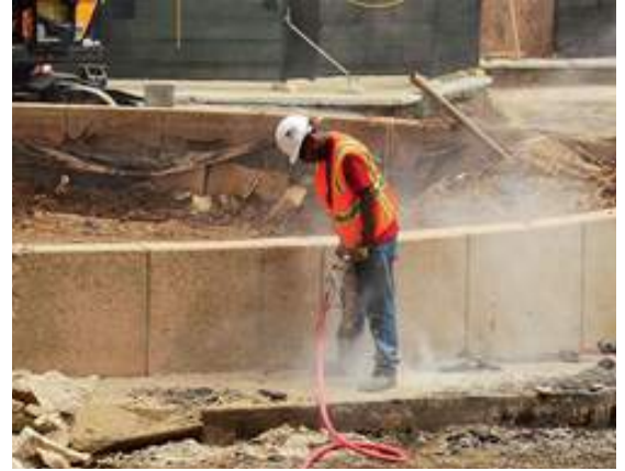
A worker breaks up concrete creating a cloud of silica dust.
