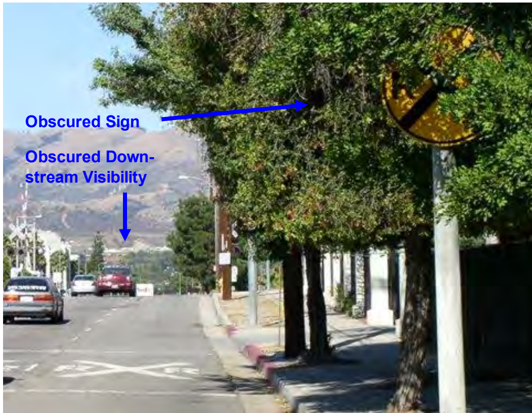
Figure 3-16. Restricted Visibility at a Highway-Rail Grade Crossing Approach
