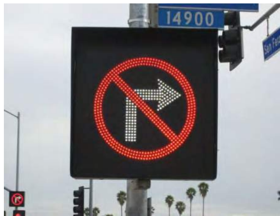
Figure 3-28. Turning Movement Blank-Out Sign
