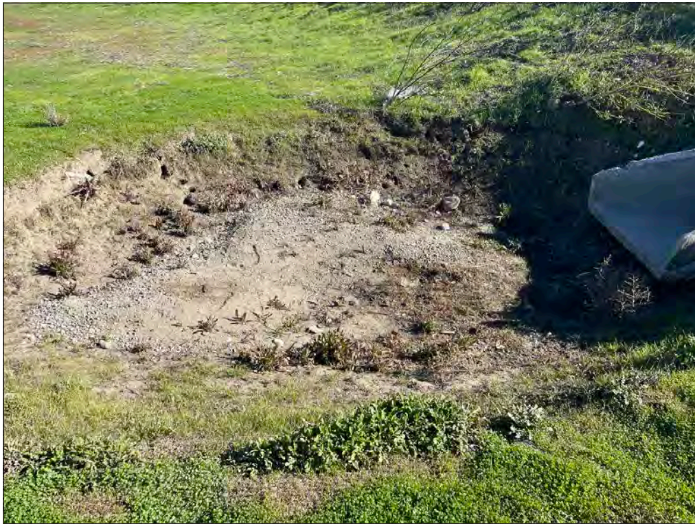
Photo 5: View of the downstream terminus of Drainage A, facing east.
