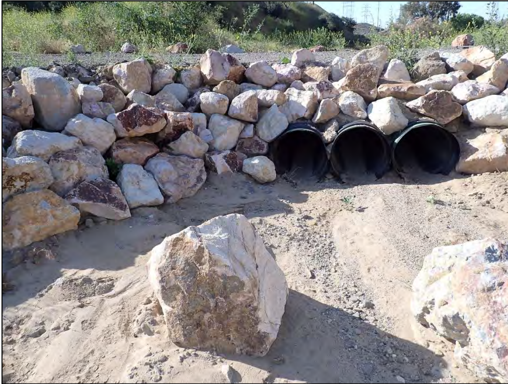
Photo 9. Culverts under road within Haskell Canyon Wash – Aquatic Feature 2; view facing south and downstream (latitude: 34.47923°, longitude: -118.5093649°)
