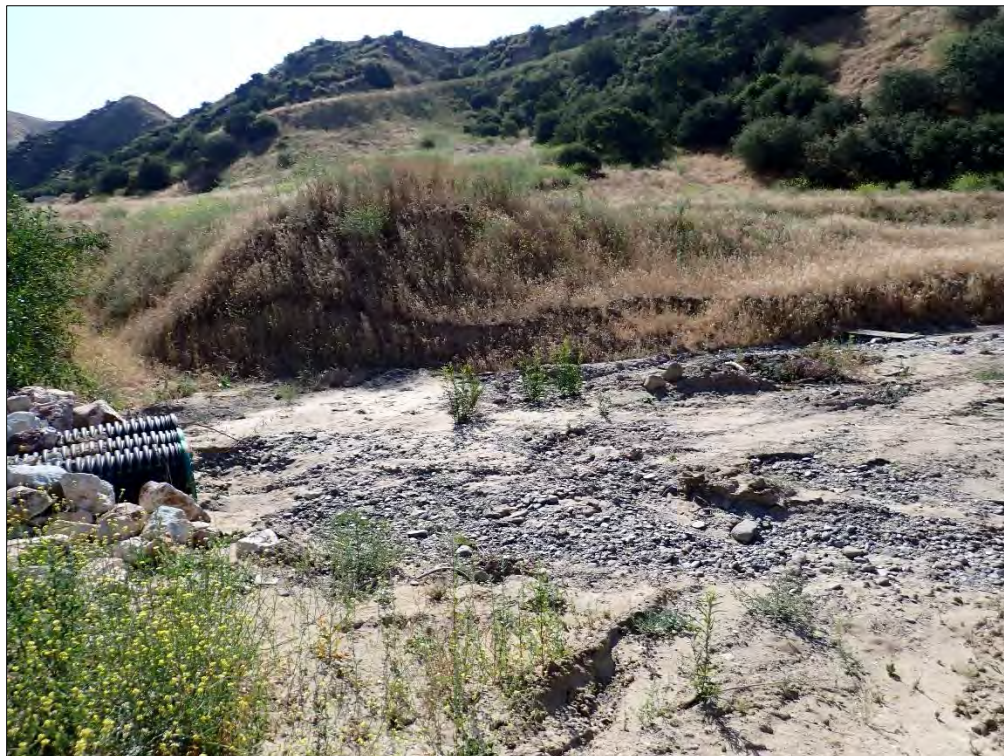
Photo 10. Culvert surfacing downstream within Haskell Canyon Wash – Aquatic Feature 2; view facing east and downstream (latitude: 34.479031°, longitude: -118.509412°)
