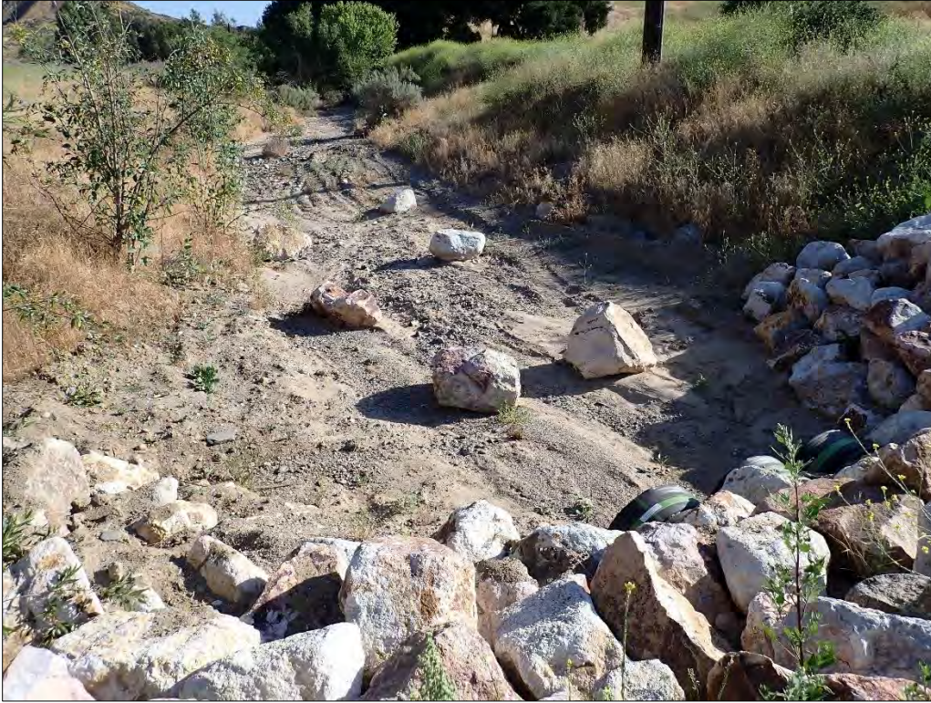
Photo 7. Haskell Canyon Wash – Aquatic Feature 2; view facing north and upstream (latitude: 34.479085°, longitude: -118.509353°)
