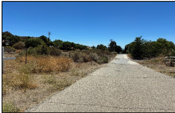
Figure 4.1-9. Lost Canyon Road at Creek Crossing; View Facing Southwest (Photo H).
