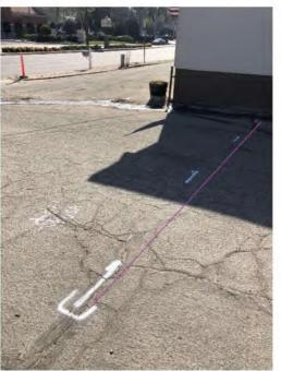
Picture 1: Linear GPR anomaly located at the driveway entrance to the parking lot. Delineated using white marking paint on site. (Purple line drawn in to visualize better)
