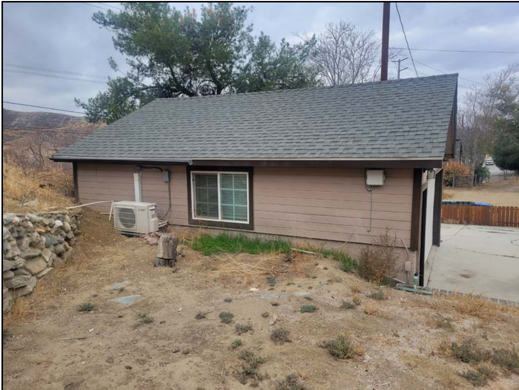
Overview of detached garage, view to the southwest. Photo # 25, 12/13/2022
