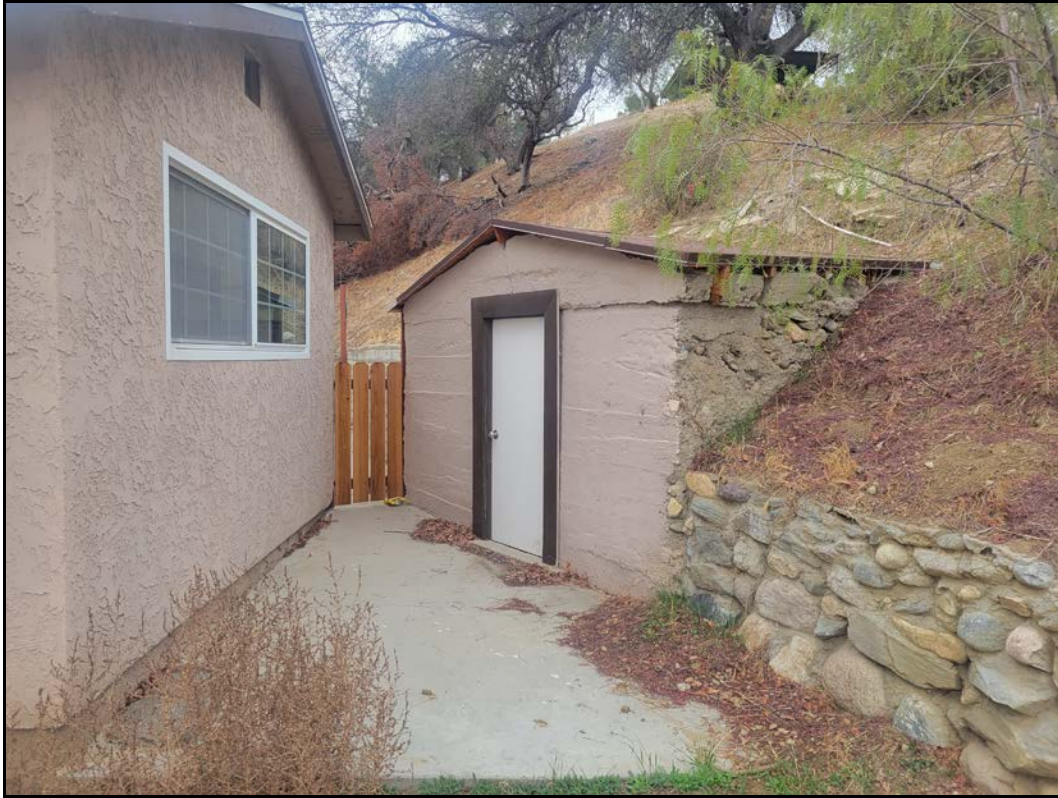
Overview of detached shed, view to the east-northeast. Photo # 23, 12/13/2022
