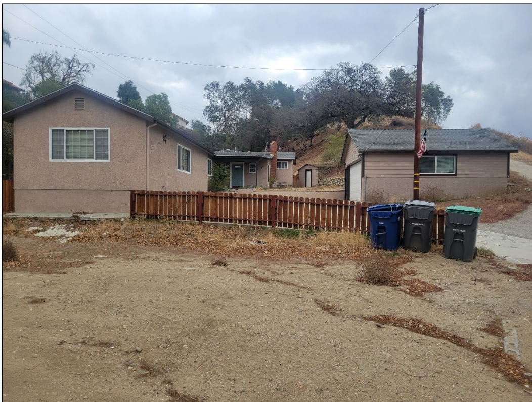
Plate 3. Overview of 28601 Bouquet Canyon Road. View to the east.
