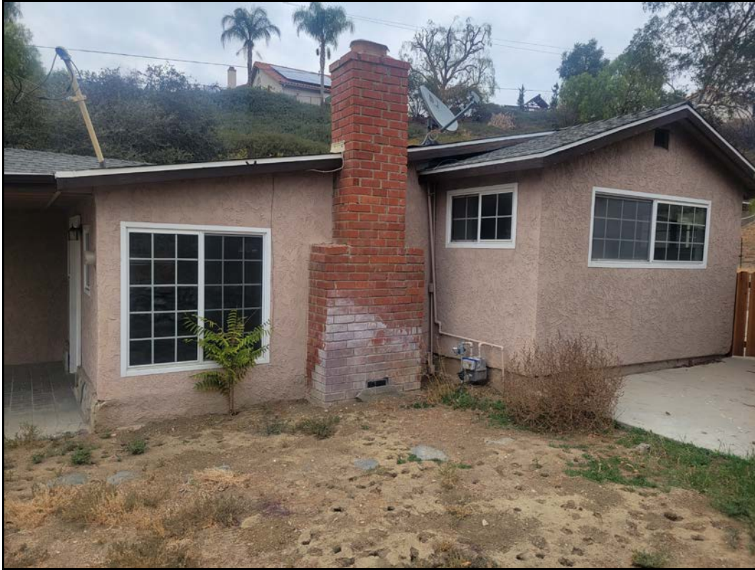
Overview of possible historic brick chimney, view to the north. Phot # 22, 12/13/2021
