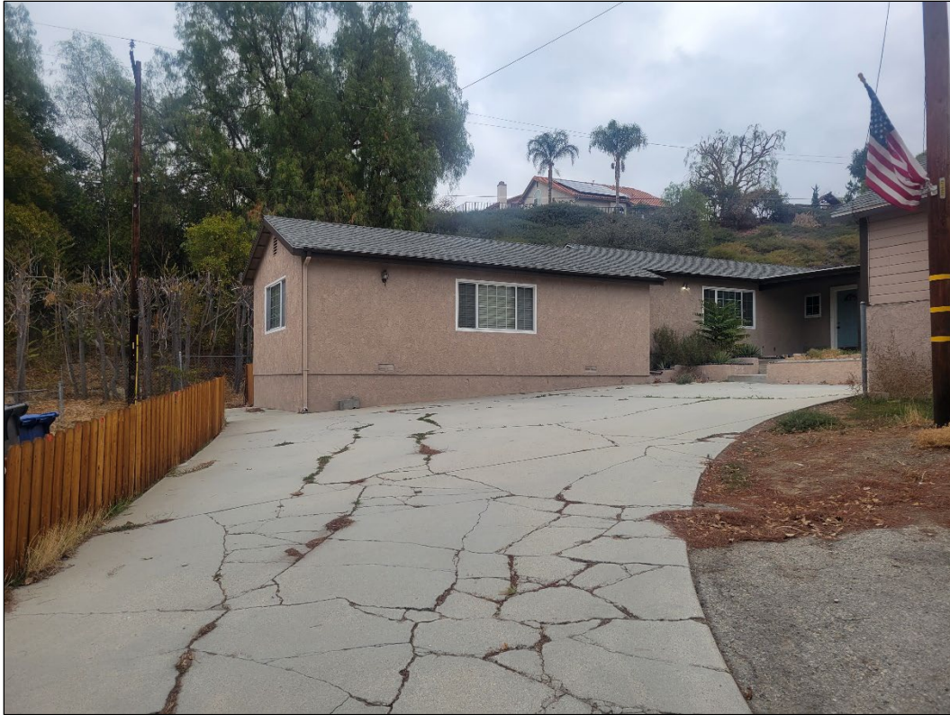
Plate 4. Overview of 28601 Bouquet Canyon Road, view to the north.
