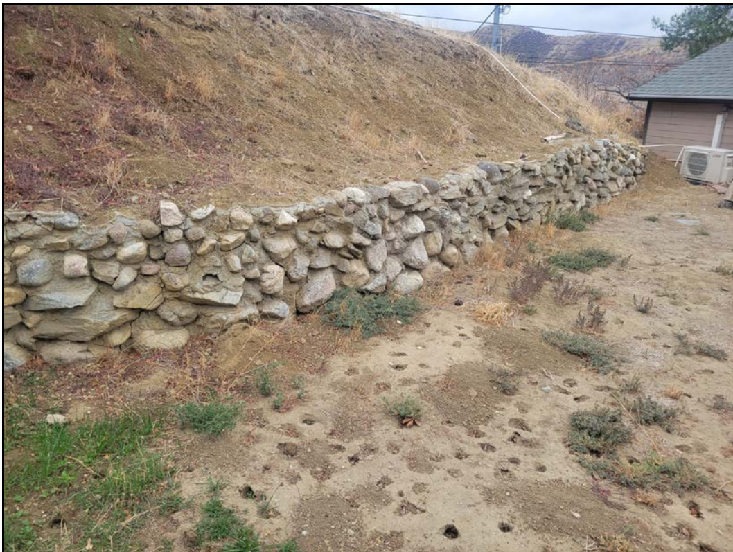
Overview of possible historic retaining wall, view to the south-southwest. Photo # 24, 12/13/2021
