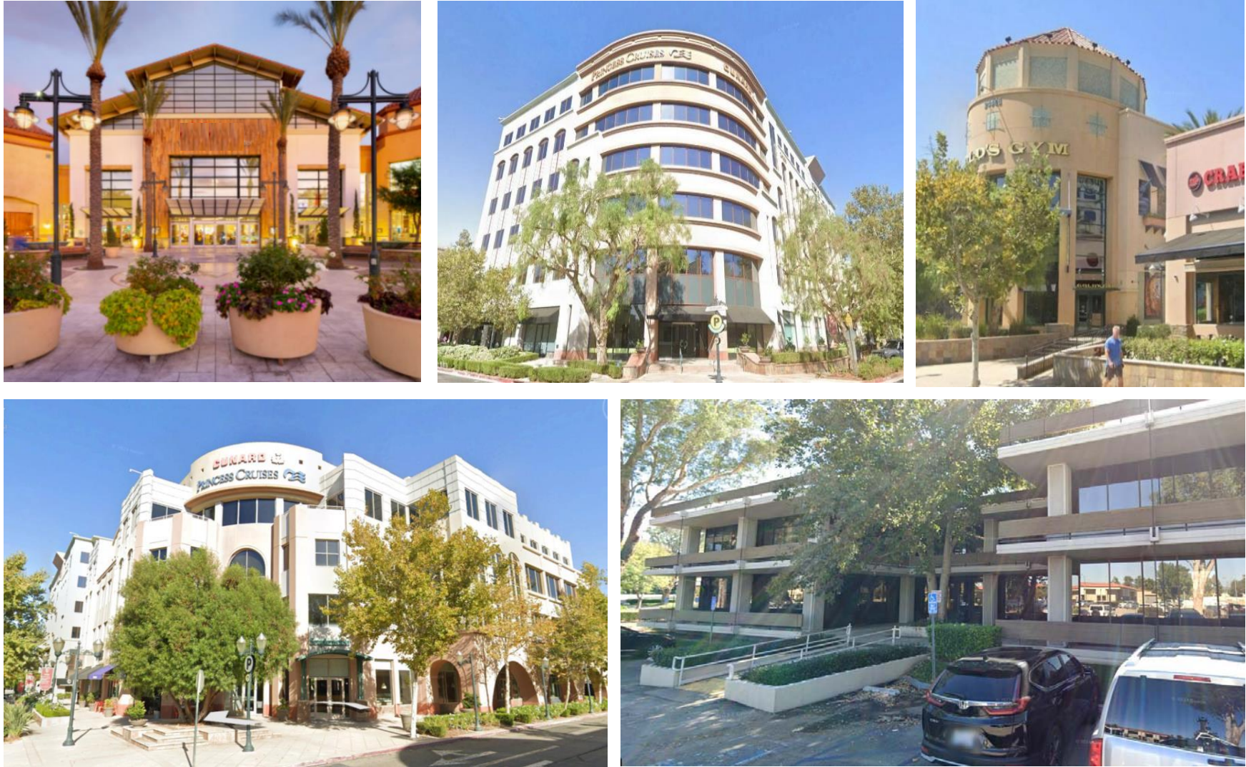
Figure 2-6. Existing Architecture in the SPA
