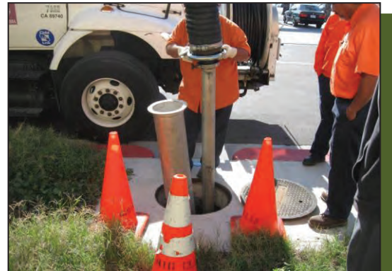
Insertion of vacuum hose into separation chamber.
