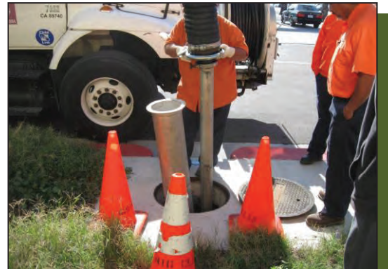
Insertion of vacuum hose into separation chamber.
