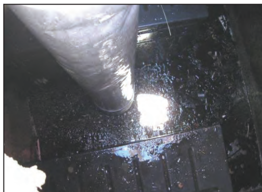
Removal of trash, sediment and debris.
