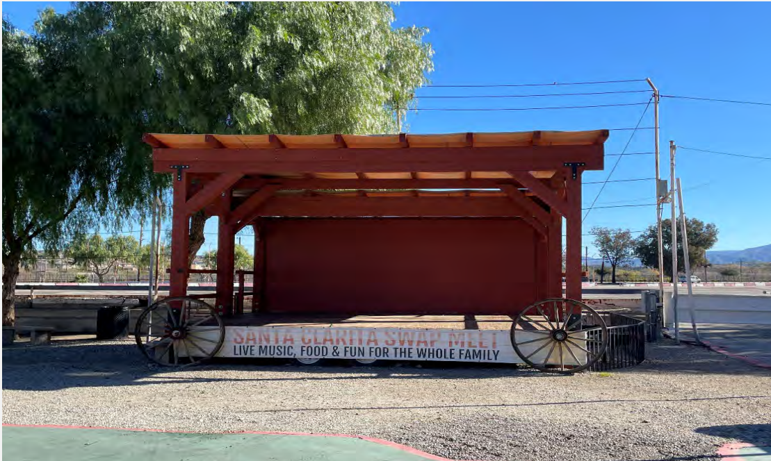
Figure 20. Overview of the Stage Platform (15), looking east (IMG_3188).
