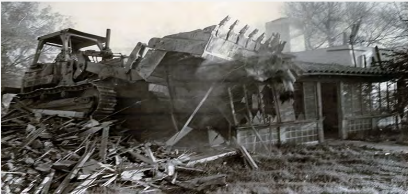
Figure 4. 1988 photo of the Baker Residence (1) being demolished (Thornhill 1988).
