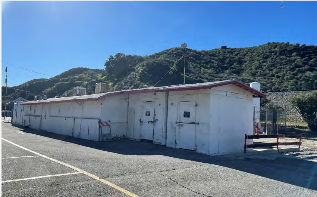
Photograph 16. Overview of the Office Building (13), view looking southwest (IMG_2047).
