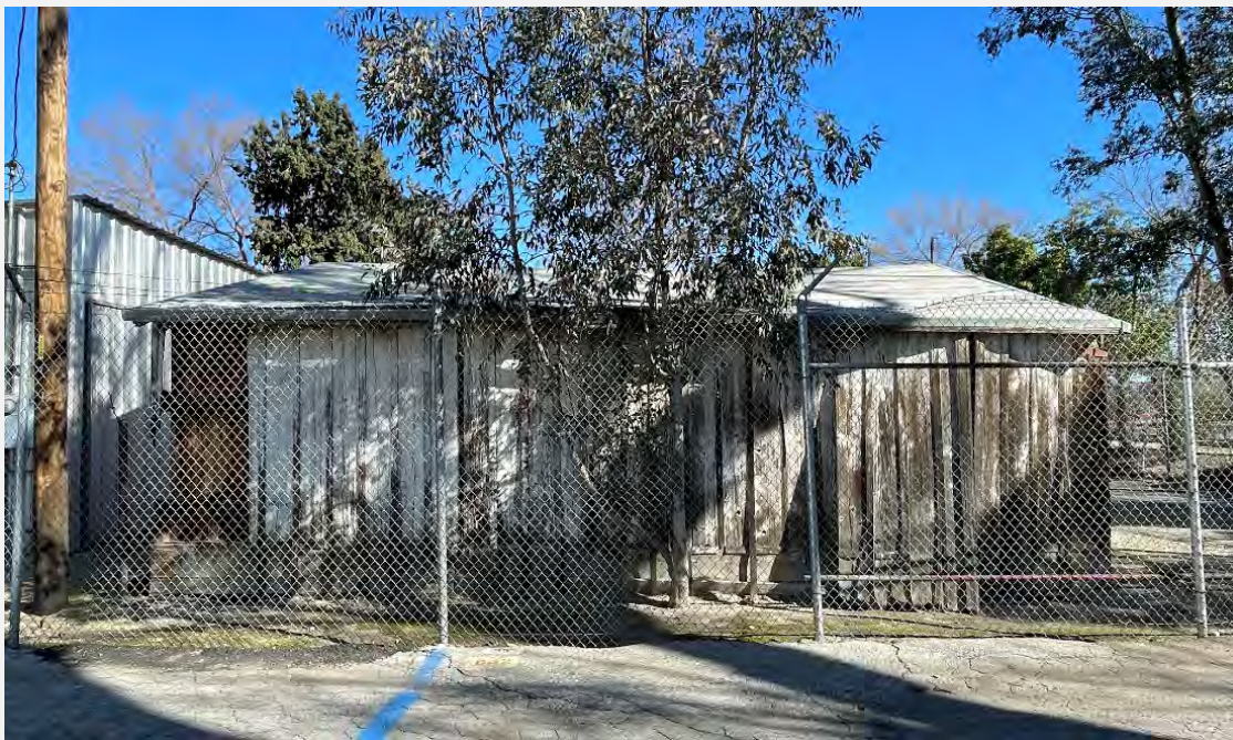
Figure 11. Overview of Ancillary Building's (8). View looking northeast (IMG_3261).
