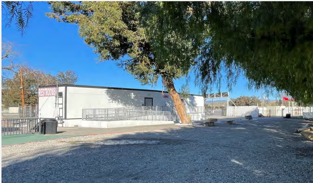
Photograph 17. Overview of the Restrooms (7). View looking northeast (IMG_3191).
