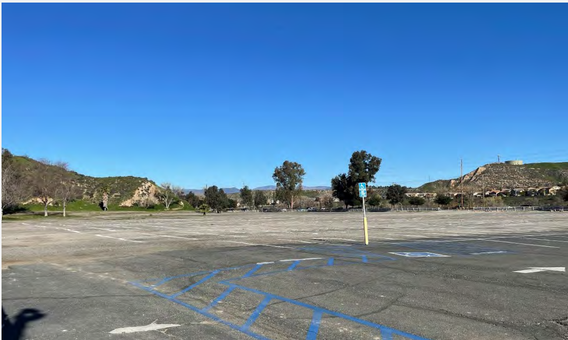
Figure 15. Overview of the Parking Lot (5) showing both the paved (foreground) and gravel (background) areas. View looking northwest (IMG_1975).
