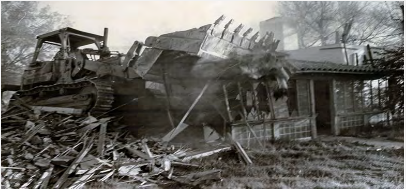
Photograph 4. 1988 photo of the Baker Residence (1) being demolished (Thornhill 1988).
