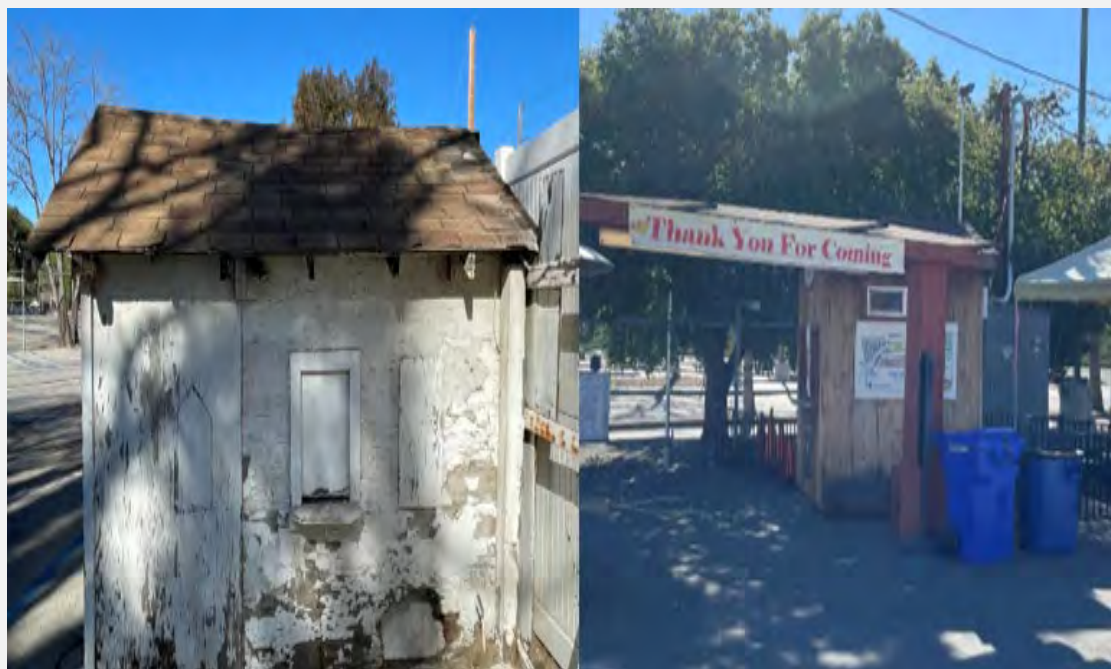
Figure 19. Overview of the two Ticket Kiosks (10), view looking east (IMG_2169 and IMG_3260).
