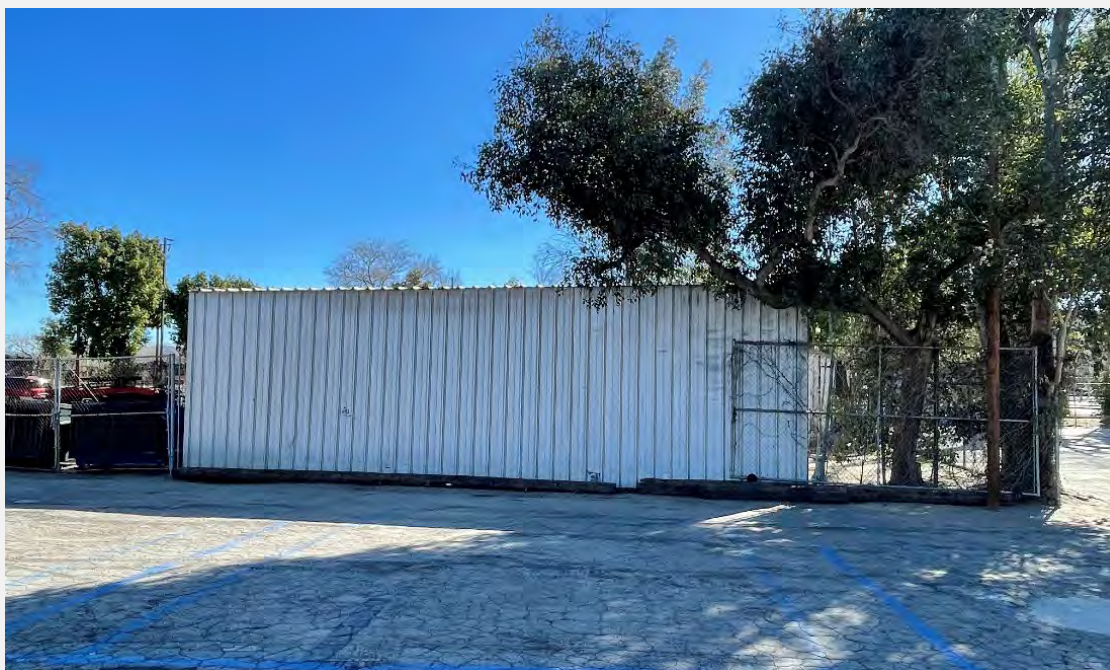
Figure 18. Overview of the Ancillary Building (9). View looking southeast (IMG_3251).
