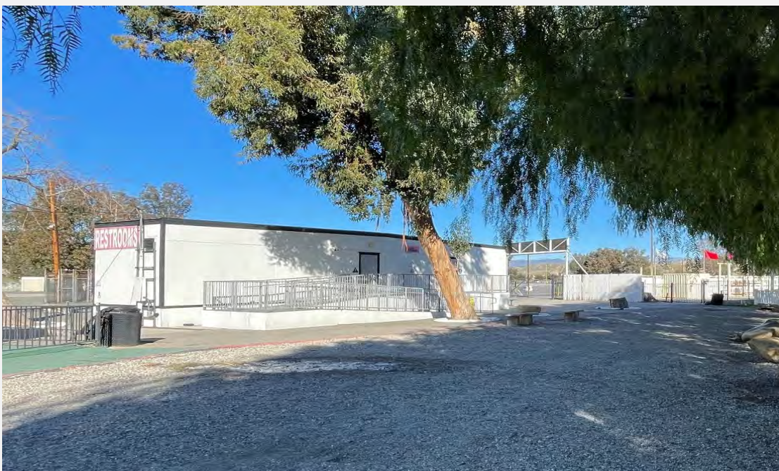
Figure 17. Overview of the Restrooms (7). View looking northeast (IMG_3191).
