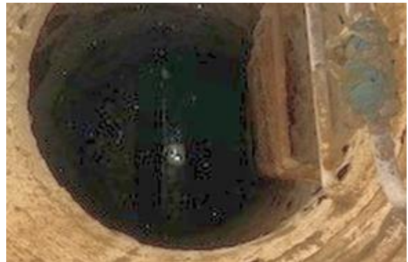
Manhole Before Install
