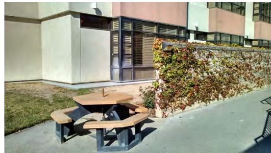
Concrete Masonry Unit Wall with Vine Coverage (Nursing Pavilion Building)
