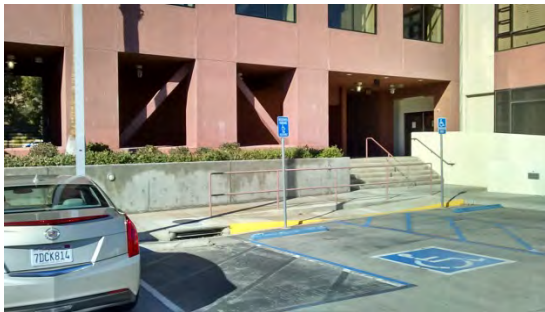
Concrete Planter (Nursing Pavilion Building)
