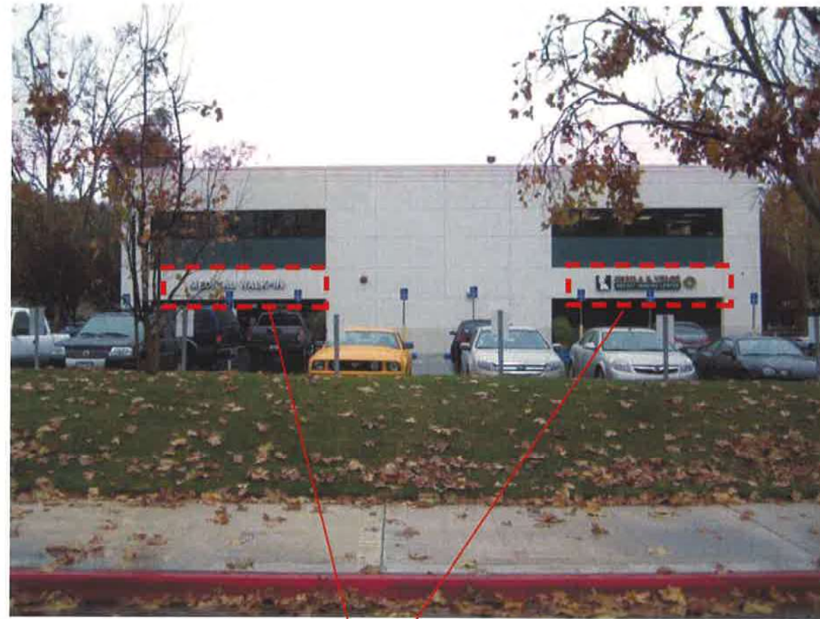
Existing Condition MOB - 23929
