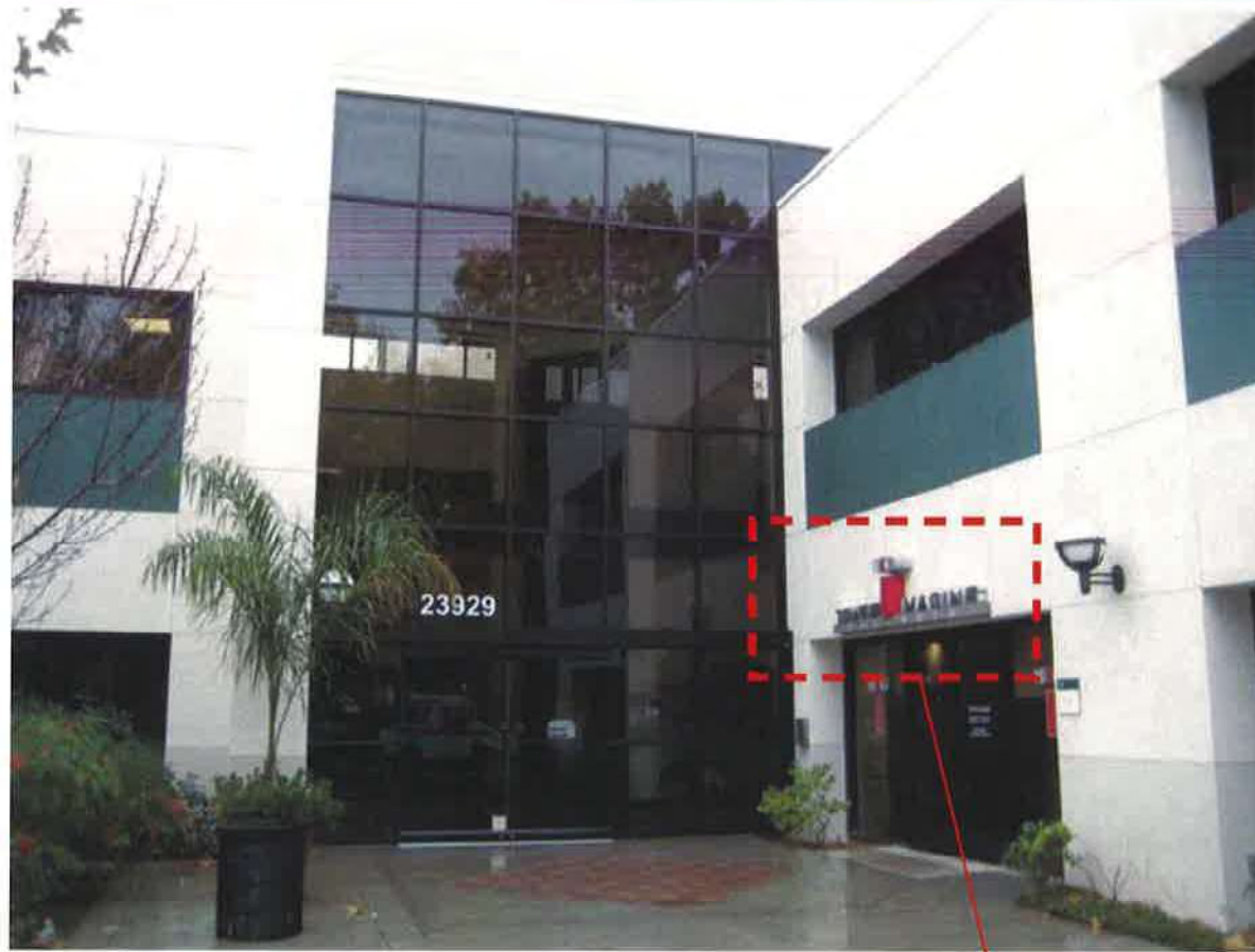
Existing Condition MOB - 23929
