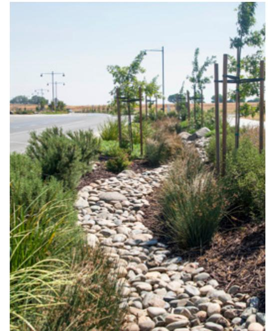
Curb side infiltration trench with meandering centerline.
