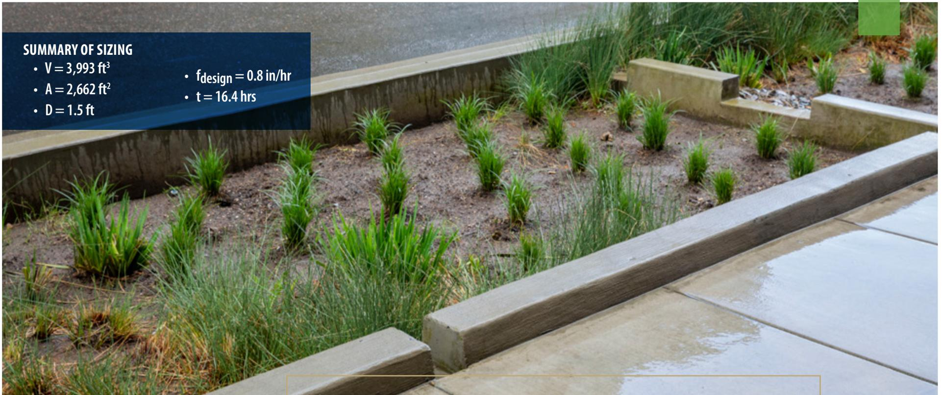
Curb side rain garden with curb slot inlets and check dams
