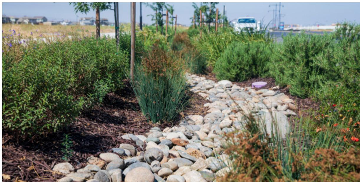
*Median infiltration trench with vegetation lined edges.*
