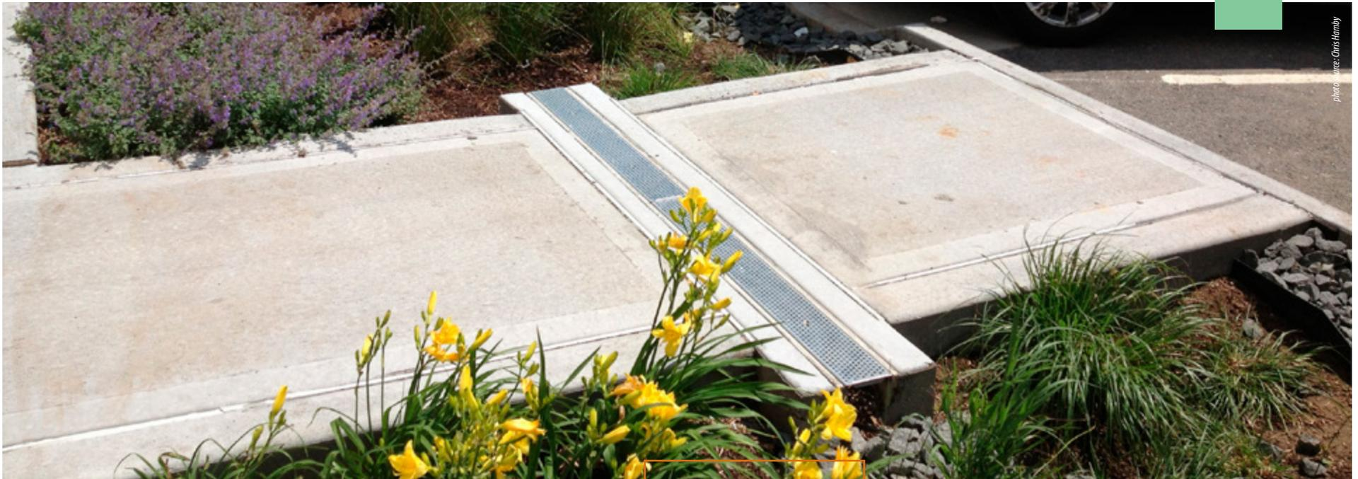
Hydraulically connected curb side rain gardens placed in series
