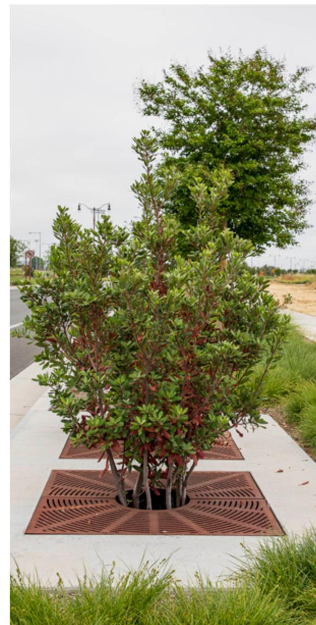
*Curb side tree box filter placed in series.*
