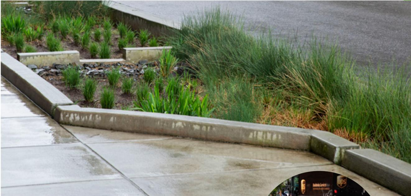
Rain gardens are vegetated areas depressed below the surrounding ground surface and surrounded by an impermeable barrier, such as a curb, with open slots that allow flow to enter. Water that enters the rain garden ponds up and slowly filters into the underlying soil, both reducing stormwater runoff volume and removing contaminants through physical and biological processes.
