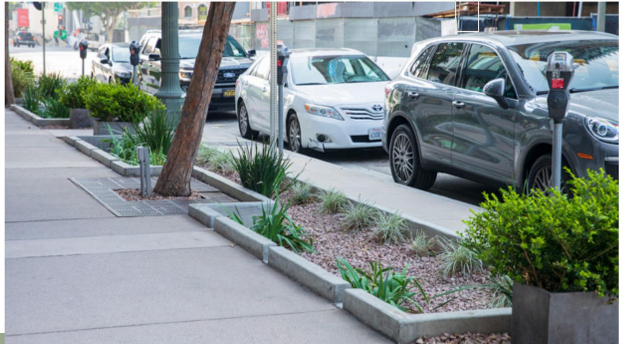
Top: Curb side rain garden with check dams and an overflow grate inlet
