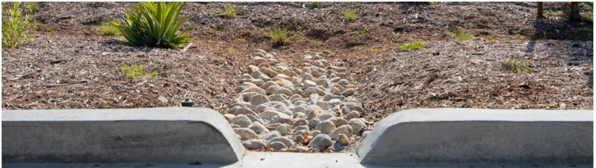
*Curb slot flow entrance with energy dissipator.*
