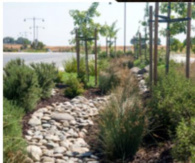
*Left: Curb side infiltration trench between sidewalk and building
