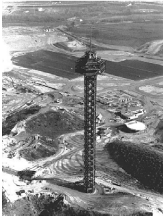
Construction of Magic Mountain-circa 1971
