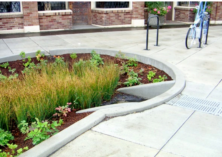
Rain gardens and bioswales help capture and filter stormwater, recharging our aquifers and improving the quality of our waterways. (Portland, OR)
