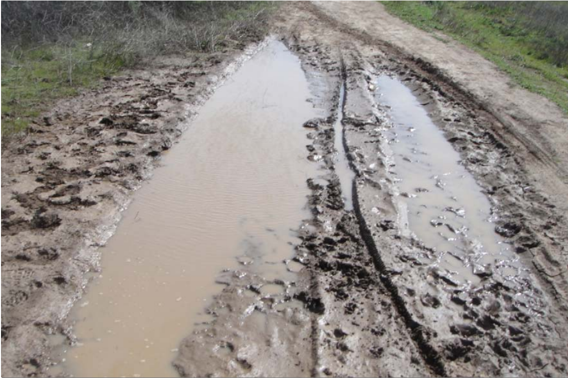
03_06_2011 Road Rut 1 : View of inundated pool within the utility access road to the south
