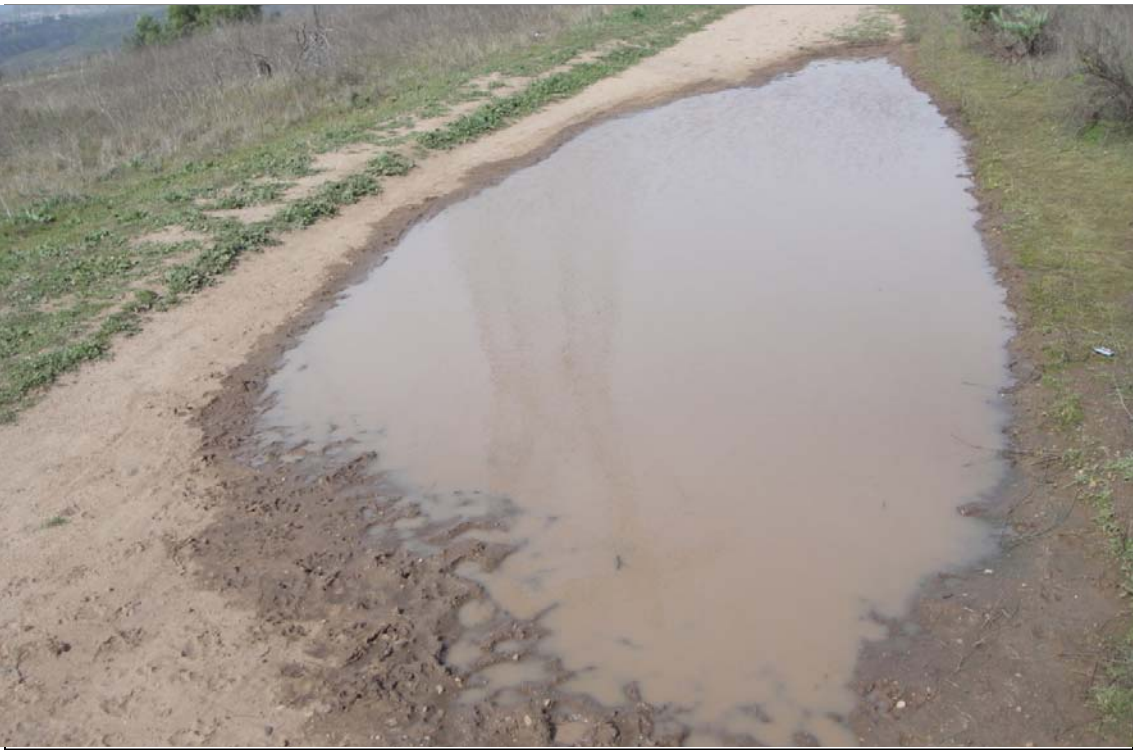
03_06_2011 Road Rut 2 : View of inundated feature within utility access road to the north.
