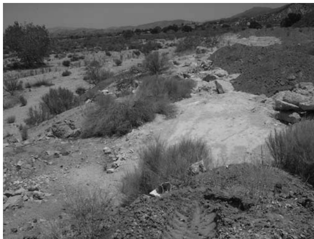
Northern Edge of Fill with Concrete
