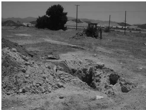
Concrete Rubble in Fill
