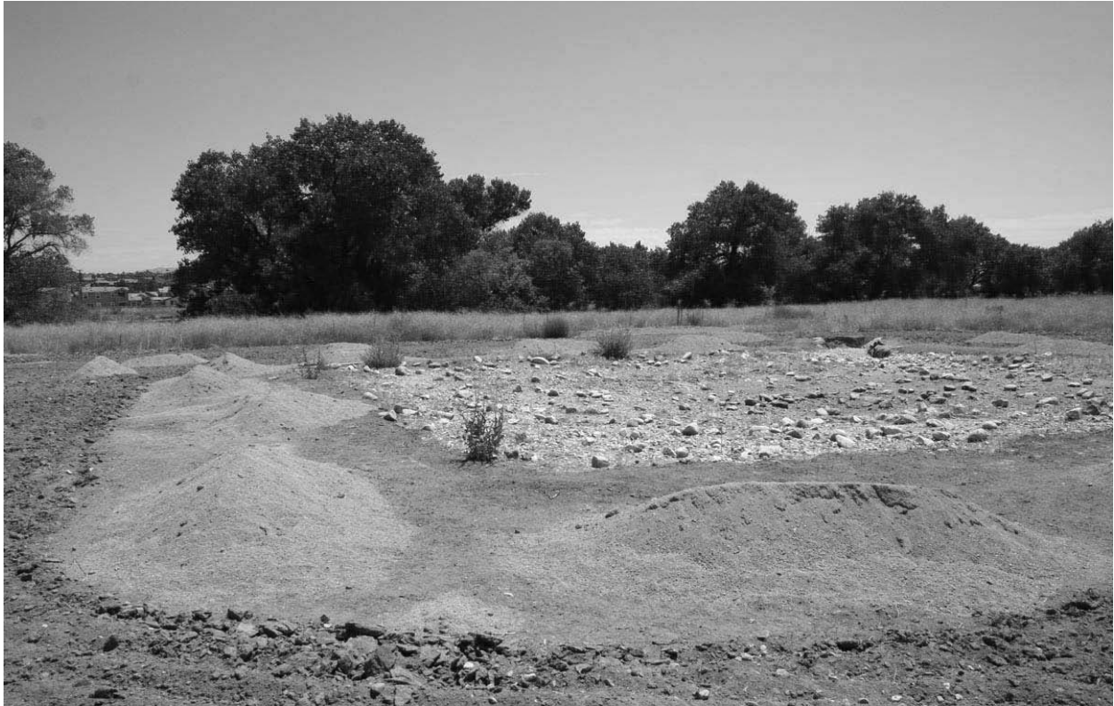
Photo 1 – View of completed Pool 1 with San Francisquito Creek in background.
