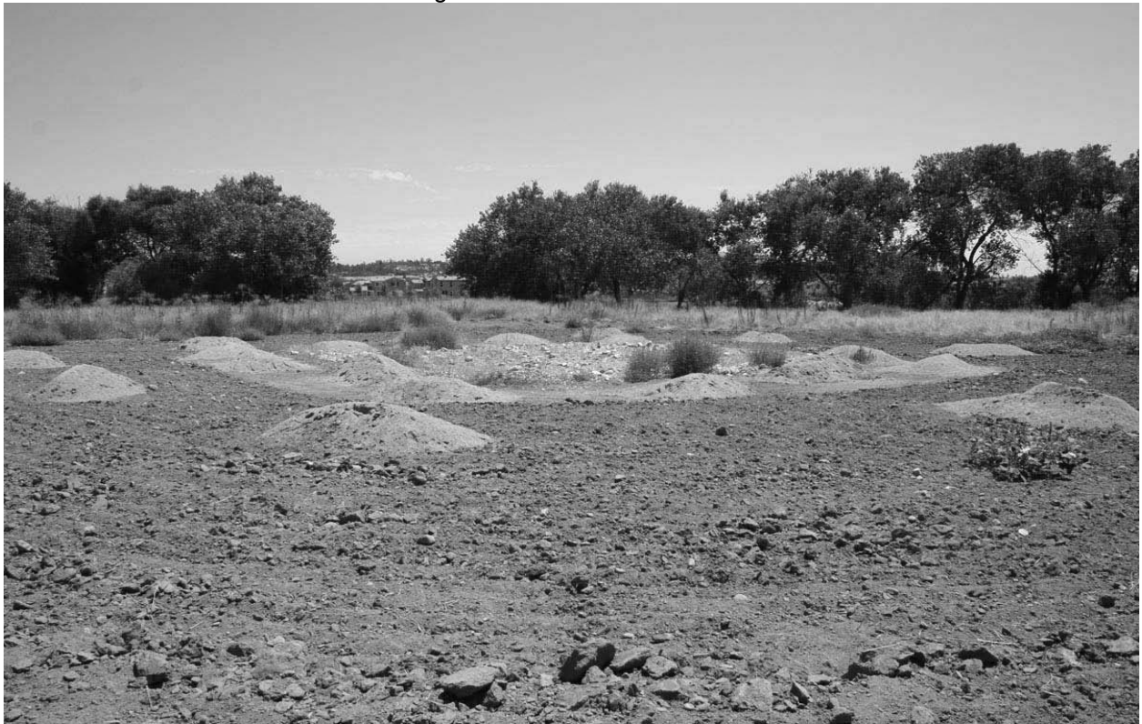
Photo 4 – View east of completed Pool 2
