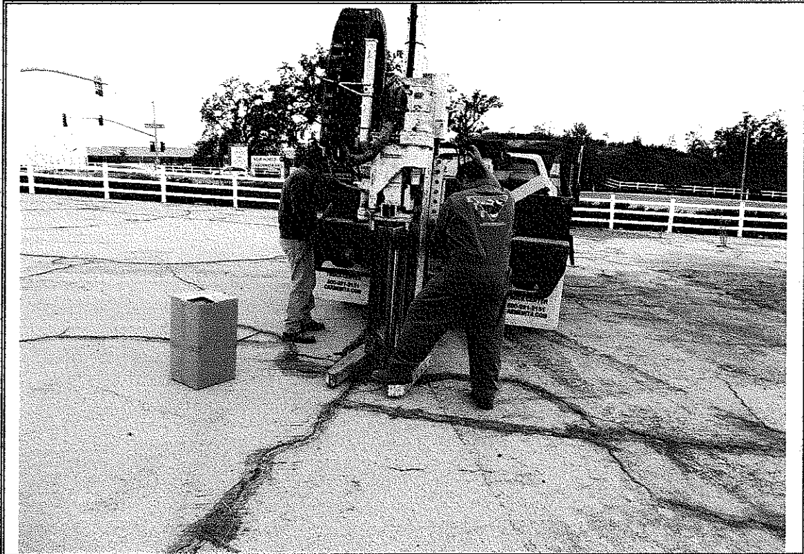
Photograph 3: View of the drilling crew installing the S1 boring.
