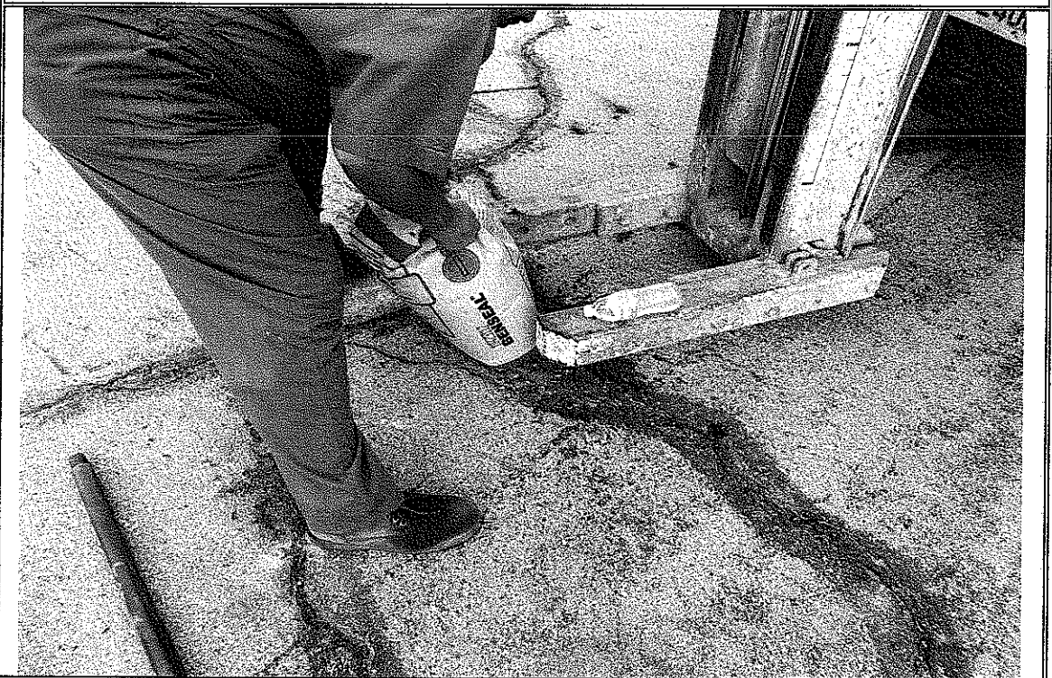
Photograph 6: View of a boring location being abandoned and plugged with asphalt.
