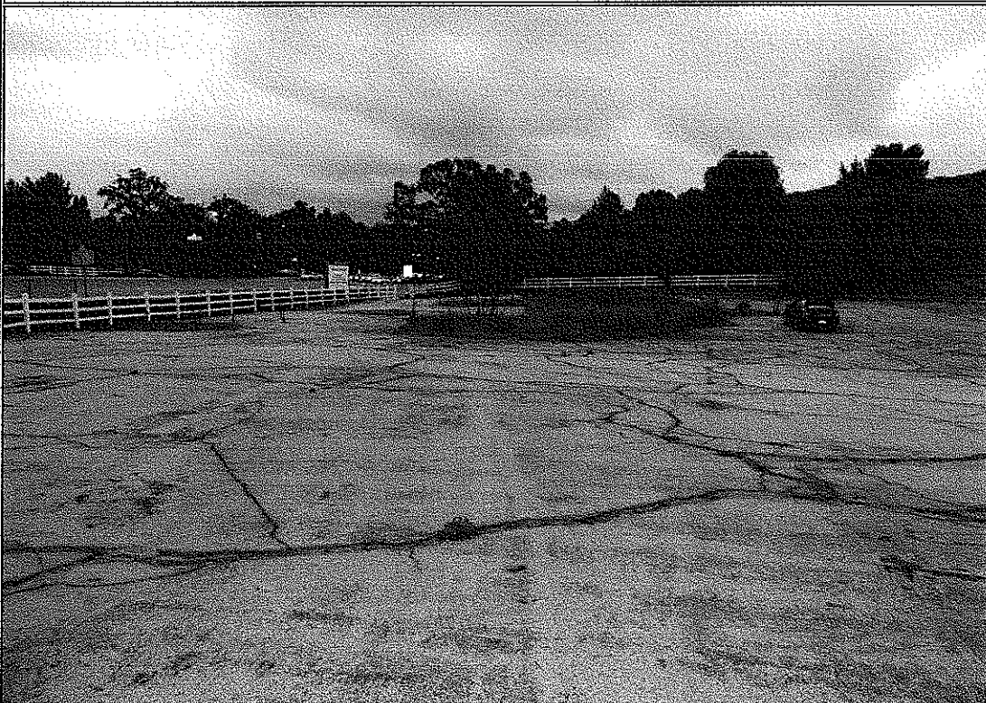
Photograph 2: View of the area of investigation looking northeast from the southwest corner of the parking lot.
