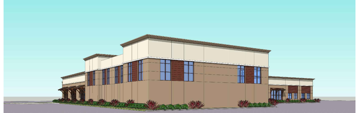
VIEW AT GYM (SOUTHWEST ELEVATION)
