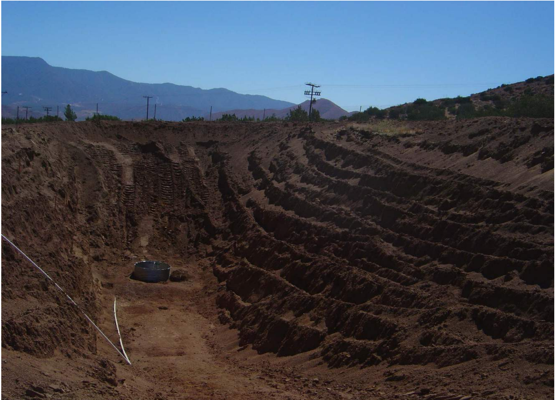
PHOTO 3–Test Basin Excavation
