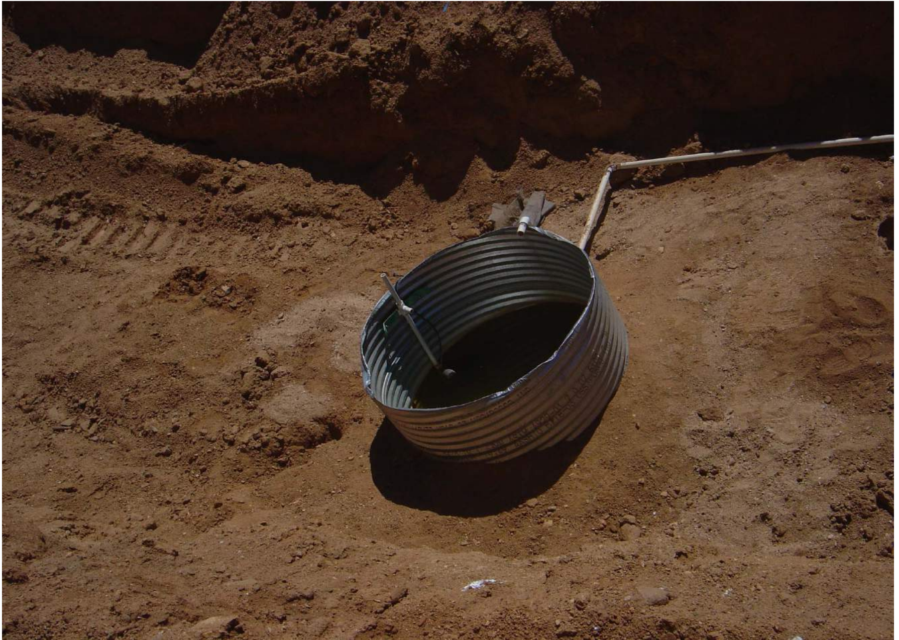
PHOTO 4–Five Foot Diameter Stand Pipe
