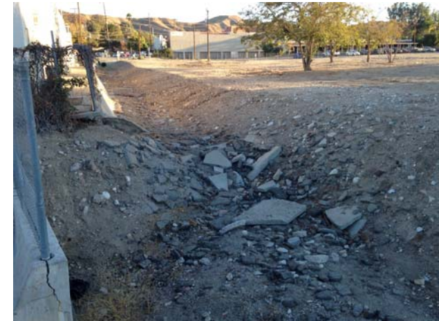
Photograph 6. View of the onsite dry Soledad Road Drainage channel with asphalt and concrete debris, facing north.
