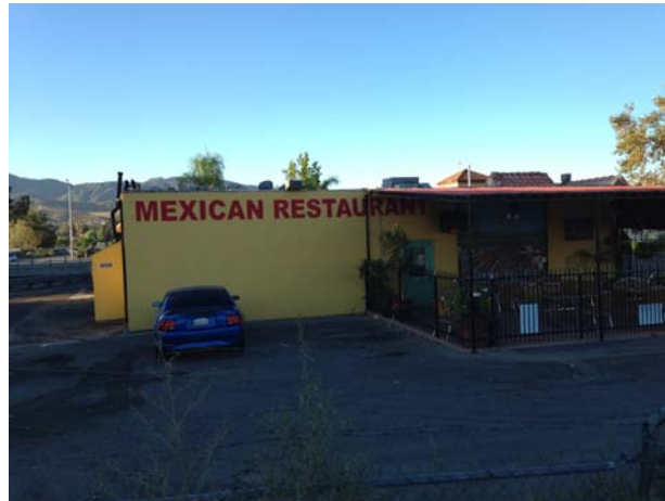
Photograph 11. View of a southern adjacent property: Casa Vieja Restaurant (18401 Soledad Canyon Road).
